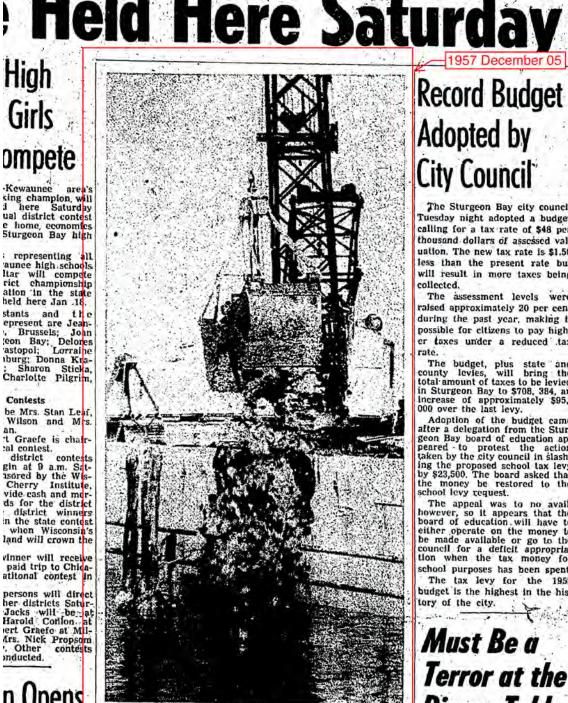
DREDGING IN REVERSE—A Roen barge was snapped filling in shoreline in front of the Door County Co-Op. Fill is carried in the barge and dumped out by the bucket. -Advocate photo
