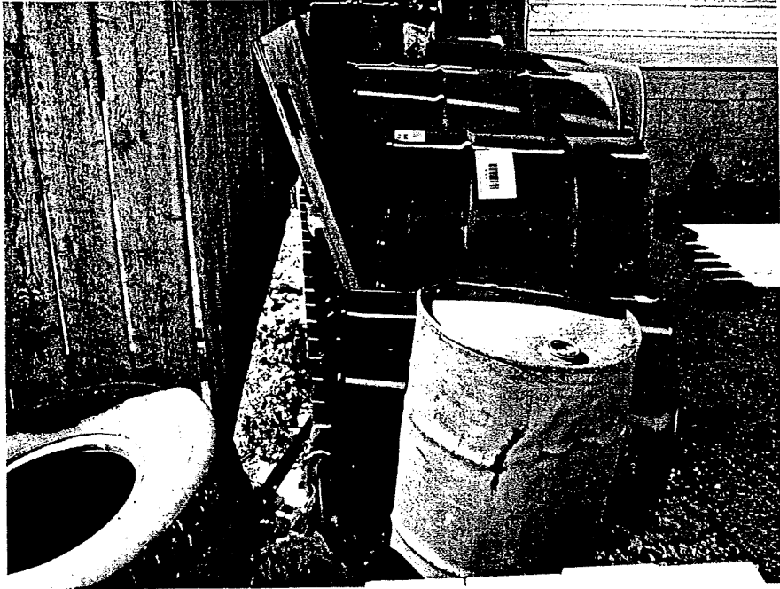
Drums and staining observed at the drum storage area.
