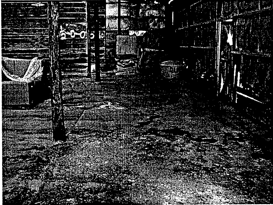
Looking west inside the northern portion of Storage Building No. 1.
