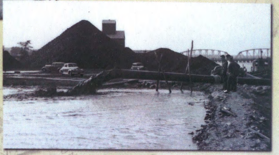
The modern dock known as Sawyer Dock was gradually lengthened by filling in the bay. Depending upon the era, the fill material may have been sawdust, garbage, or dredged material. This photo shows the dock being extended around 1940 when it was known as the Bushman Dock. Dredged material is being pumped from the shipping channel into the area behind a newly established shoreline. The photo looks northerly with the Michigan Street Bridge in the background.
