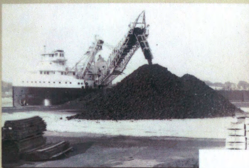
The modern dock known as Sawyer Dock was gradually lengthened by filling in the bay. Depending upon the era, the fill material may have been sawdust, garbage, or dredged material. This photo shows the dock being extended around 1940 when it was known as the Bushman Dock. Dredged material is being pumped from the shipping channel into the area behind a newly established shoreline. The photo looks northerly with the Michigan Street Bridge in the background.
